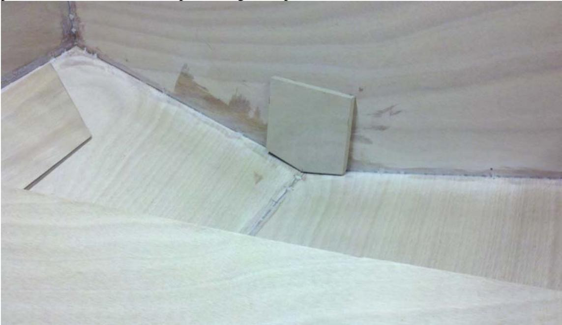
Measure three inches forward of the rudder backing plate and place a piece of tape. Do not make a pencil mark. Trim the rear flotation tank until it perfectly fits the transom and glue into place using staples or small tack nails.
